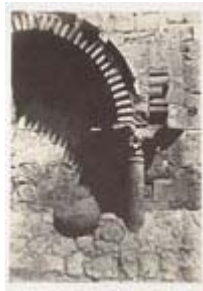
Fig. 9 Auguste Salzmänn, photographer: western portal, Church of the Holy Sepulchre, Jerusalem, 1854, salted paper print, 33.0 x 23.5 cm, PH1979:0085, Collection Centre Canadien d'Architecture / Canadian Centre for Architecture, Montréal
